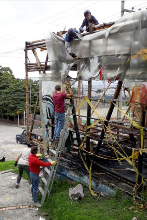
Figure 4: Casa del Viento disassembling process. Source: Own elaboration, 2017.
